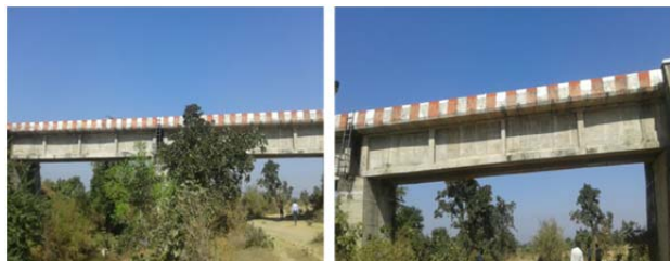
Fig. 5.1 Photograph sample of Railway bridge
